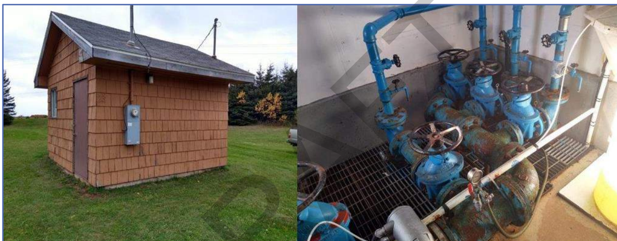
Figure 1. Pump house, containing main manifold, electronic controls, chlorine equipment and manifold inside the pumphouse
