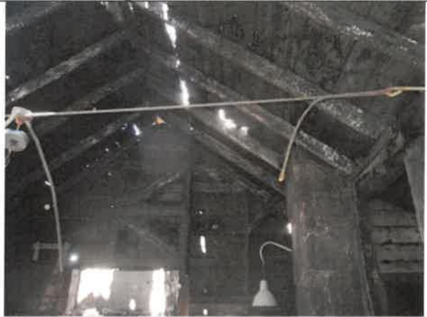
Photo #4: A view of the interior of the building showing fire damaged roof rafter and wall studs.
