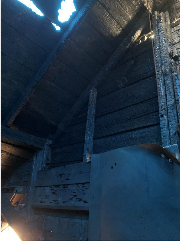
Fire Damage of Exterior West Wall
