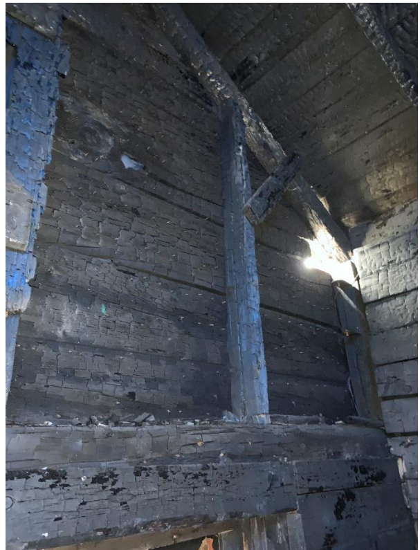
Fire Damage of Exterior East Wall
