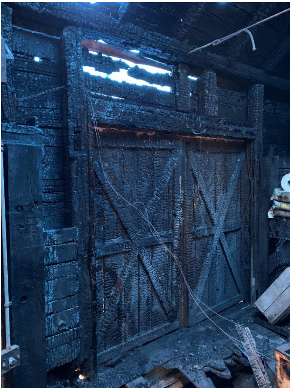
Fire Damage along North Wall
