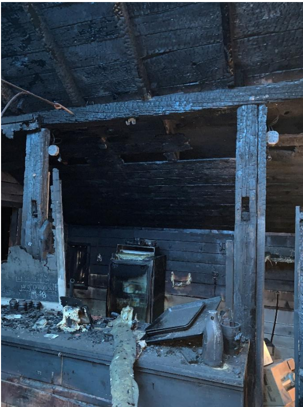
Fire Damage of Interior Support Columns & Beams
