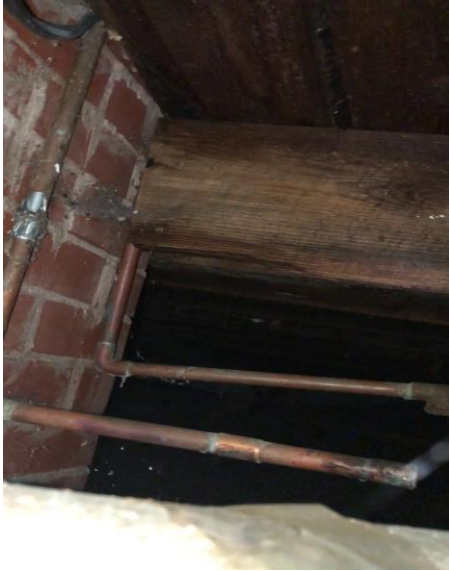
Photo 19: Joist with no end support.
