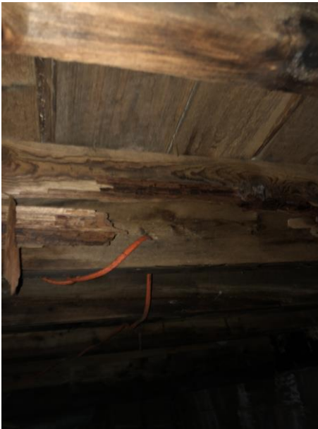
Photo 14: Severely rotted joists
