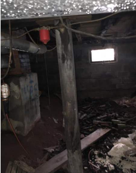
Photo 13: Condensation build up on the ducting above. Undermined chimney foundation.
