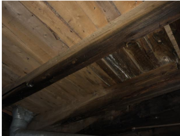
Photo 16: Severe rot in joists and deck planks.
