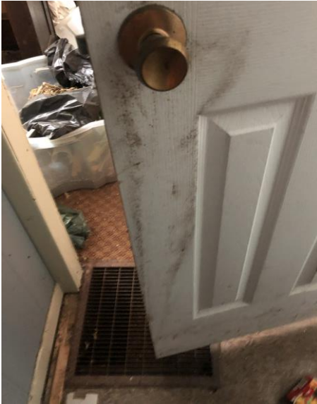
Photo 9: Suspected mold growing on living room door.
