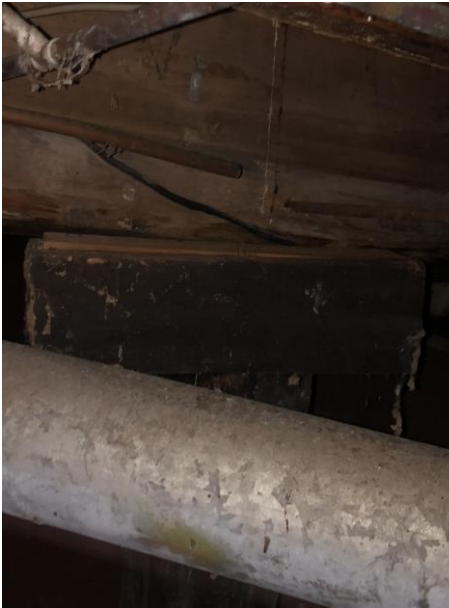
Photo 20: Beam post with no bearing.
