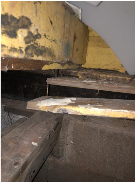
Photo 26: Stair landing unsafe to carry load.
