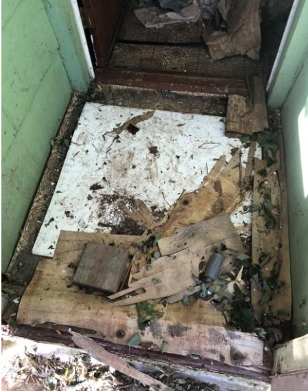
Photo 3: East Porch – Rotted floors and debris collecting.
