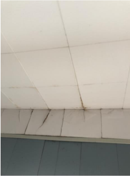
Photo 7: Water staining in ceiling near front porch.
