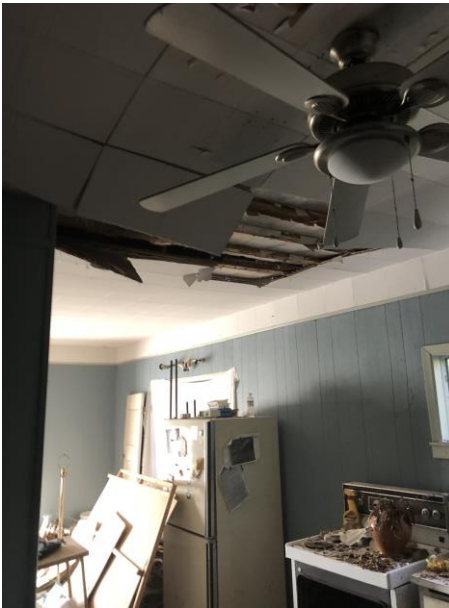
Photo 6: Exposed ceiling joists over kitchen area.
