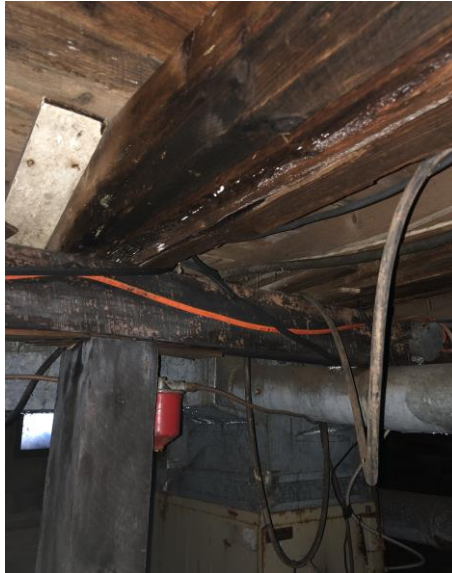
Photo 15: Severely rotted joist.
