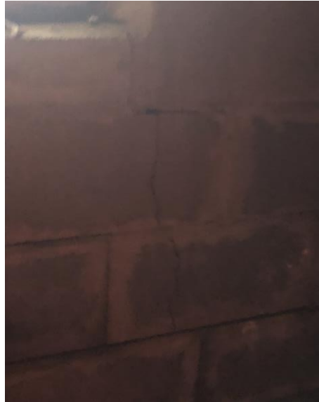
Photo 21: Wide crack in west side block wall.
