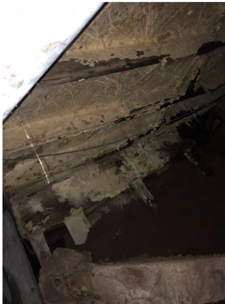
Photo 18: Unknown film/build up over approximately 10 m 2 in north east – north center floor area.
