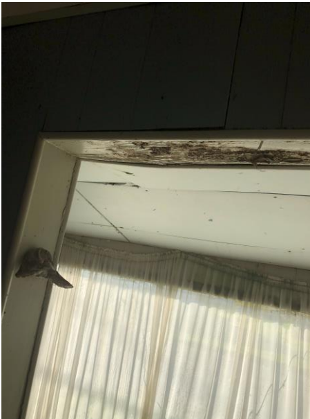
Photo 8: Severely rotted door frame with fungus growth at front porch.
