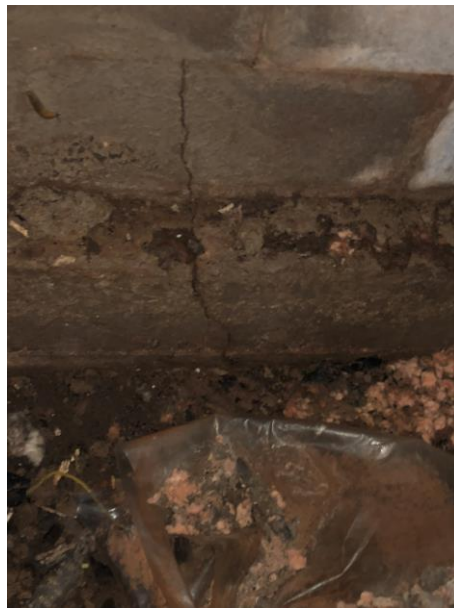
Photo 24: Wide crack through exposed wall footing.
