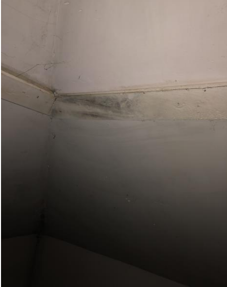
Photo 11: Suspected mold in 2 nd floor back room.
