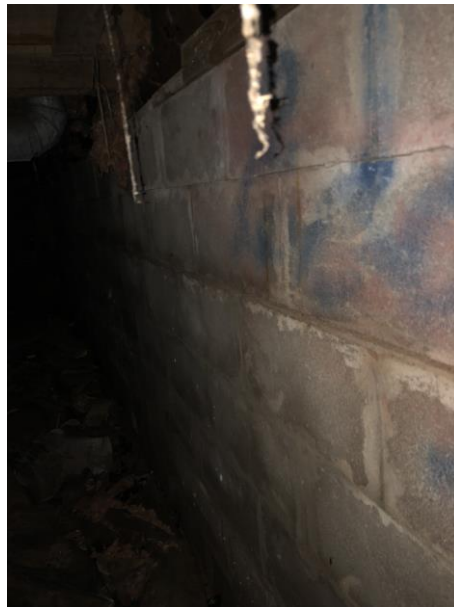
Photo 22: Wide cracks in longitudinal grout lines.
