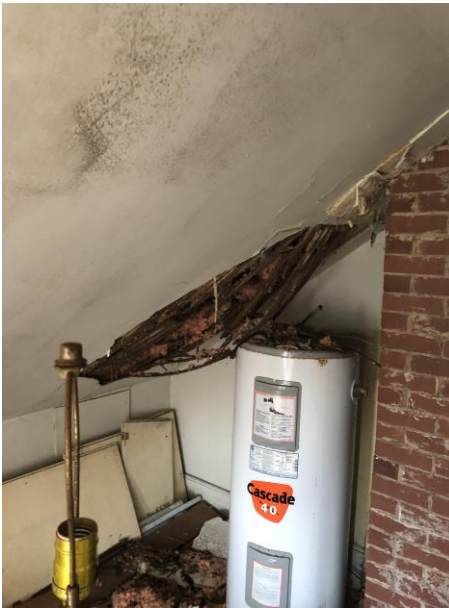
Photo 10: Collapsed ceiling due to severe rot. Large areas of mold growth/
