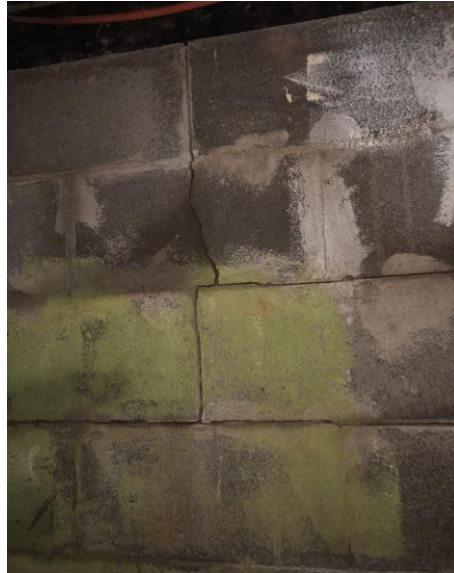
Photo 23: Wide cracks in north wall grout lines. One crack through the middle of block (2 nd course from top).
