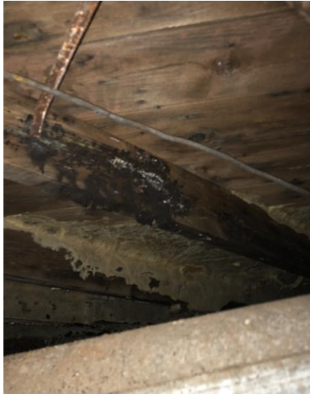
Photo 17: Rot and mold build up on joist.
