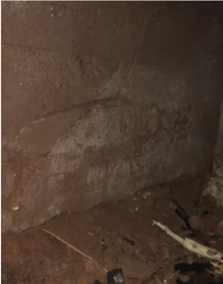
Photo 25: Wide cracks in poured wall section.
