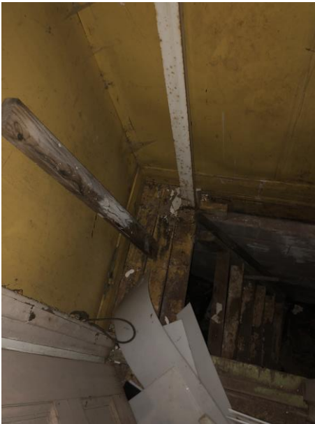
Photo 12: Basement stairs in poor condition, unsafe for use.
